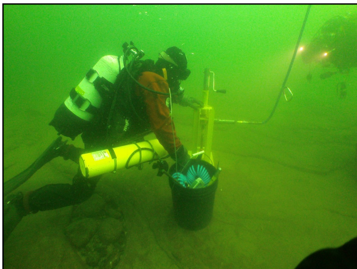
Diver setting up rock drill for anchor bolts.
