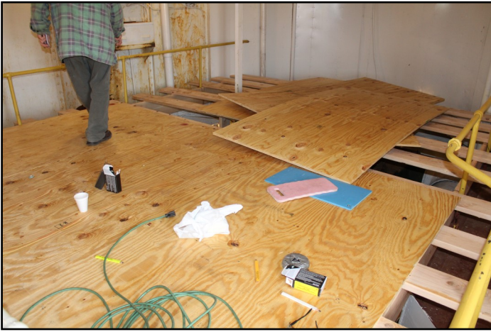
Platform above engine for ceiling work.
